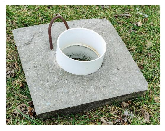
1500 GALLON TANK OR 1000 GALLON SEPTIC TANK ACCESS LID WITH 6" PVC COUPLING
